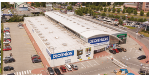
Retail Arena CHODOV
