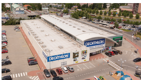
Retail Arena CHODOV
