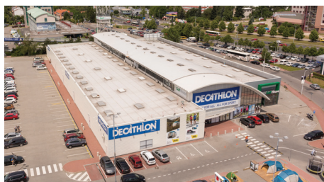
Retail Arena CHODOV
