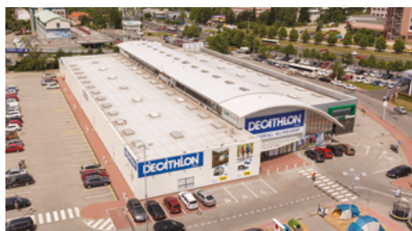
Retail Arena CHODOV
