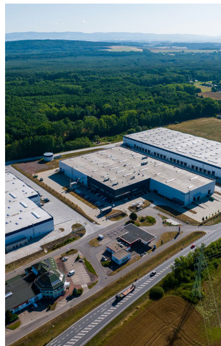
Logistic park Týniště II. a III.
