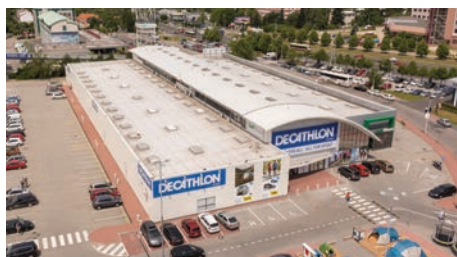
Retail Arena CHODOV
